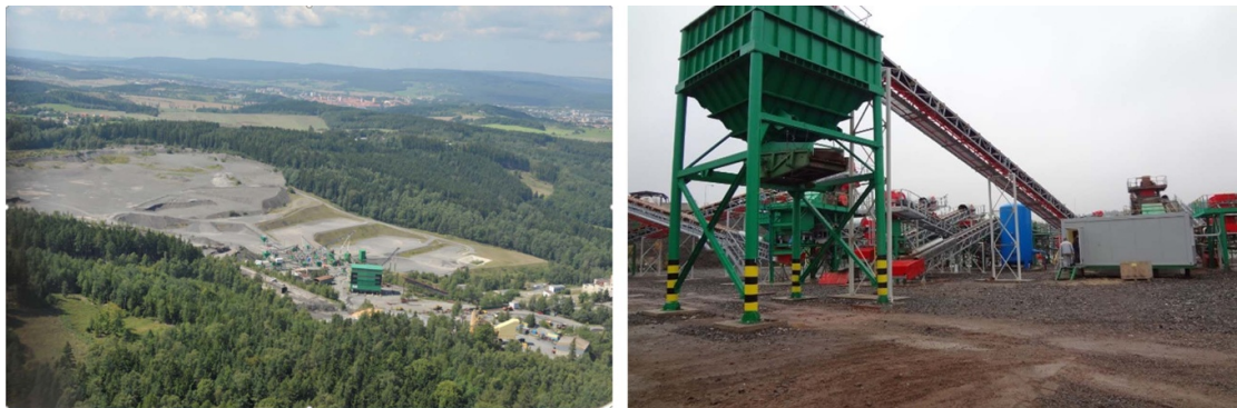
Figure 17. Site and equipment for extracting and sorting aggregates.
