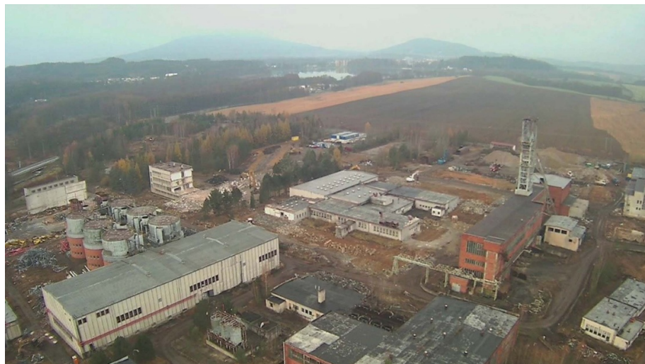
Figure 6. Mine Hamr I surface compound decommissioning.
