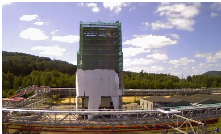
Figure 7. Uranium concentrate dryer building.
