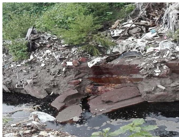
Fig. 4. Note the constant runoff of leachates, these could impact on groundwater
