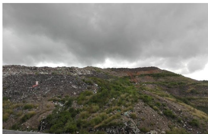
Fig. 1. A mountain of trash with dirt and leachate on top
