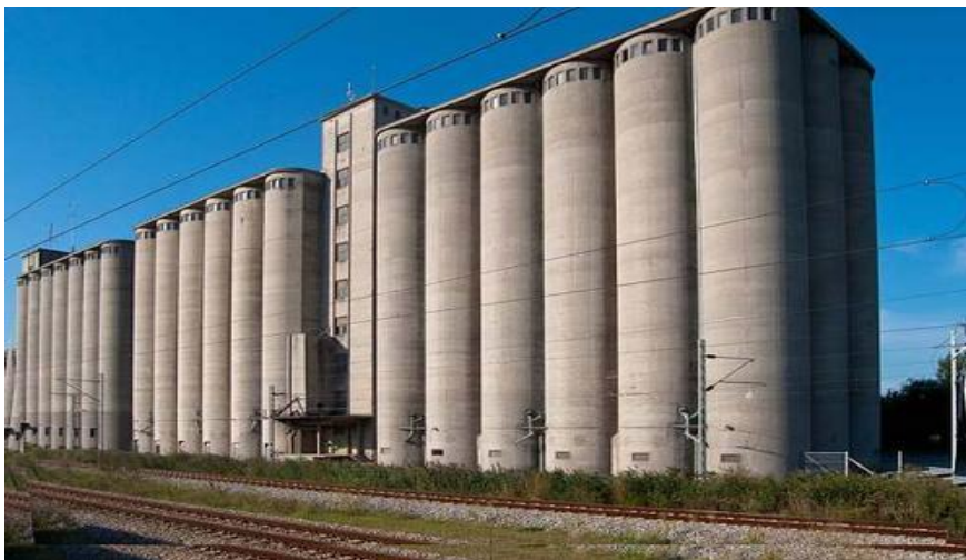
Fig. 1. Reinforced concrete silo
